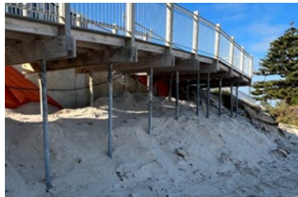
Normanville SLSC retaining wall
