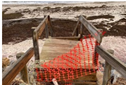
Myponga Beach stair access
