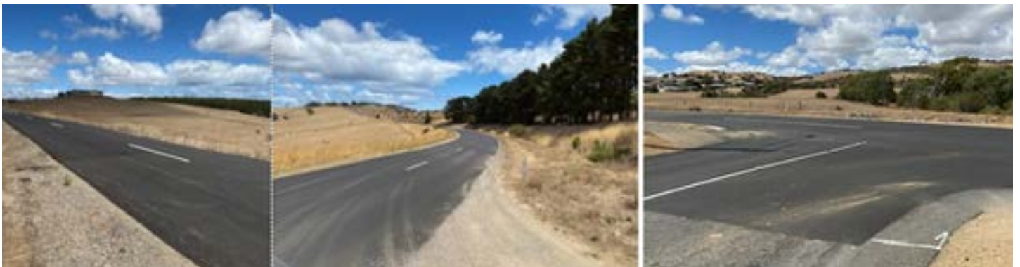
Sealed Road Program
