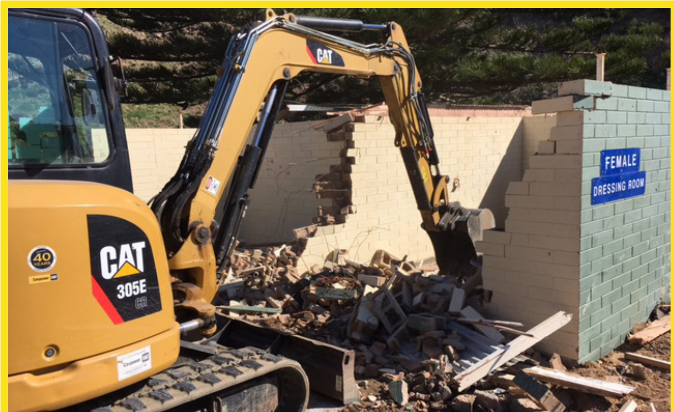
Image: Second Valley Toilet Block Demolition
