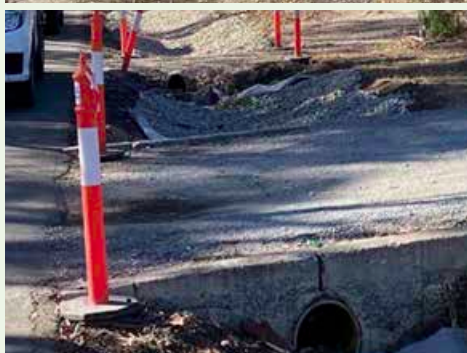
Finniss Vale Drive – Construction Underway
