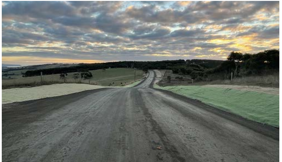
Sealed Road Program
