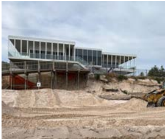
Normanville foreshore retaining wall sand shaping
