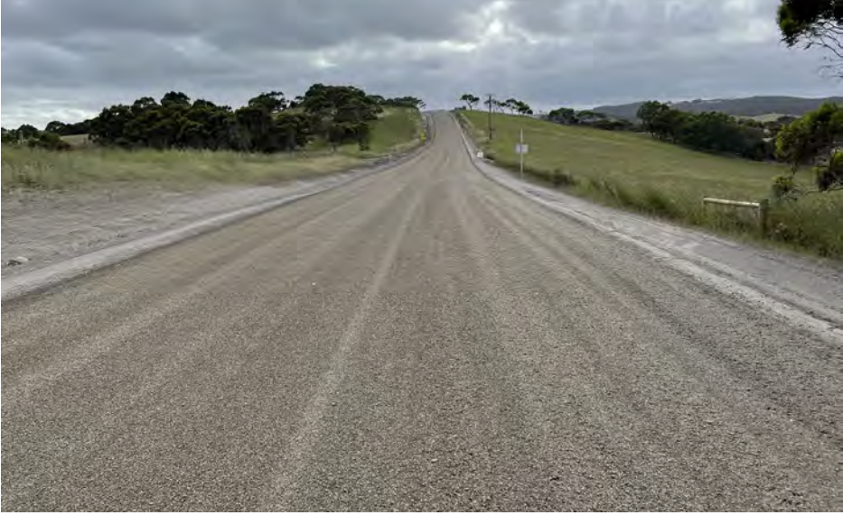
Fork Tree Road sealing
