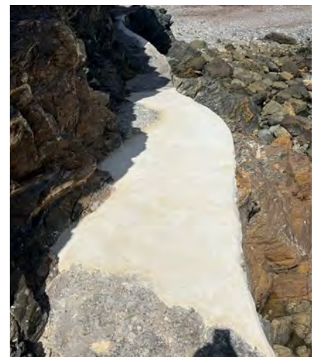
Second Valley Cliff Pathway Repairs
